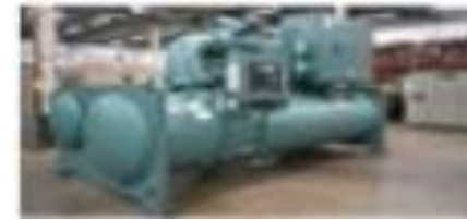
Water Cooled Chiller 0.53 IKW/TR
